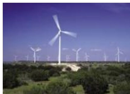
Power generation and distribution
